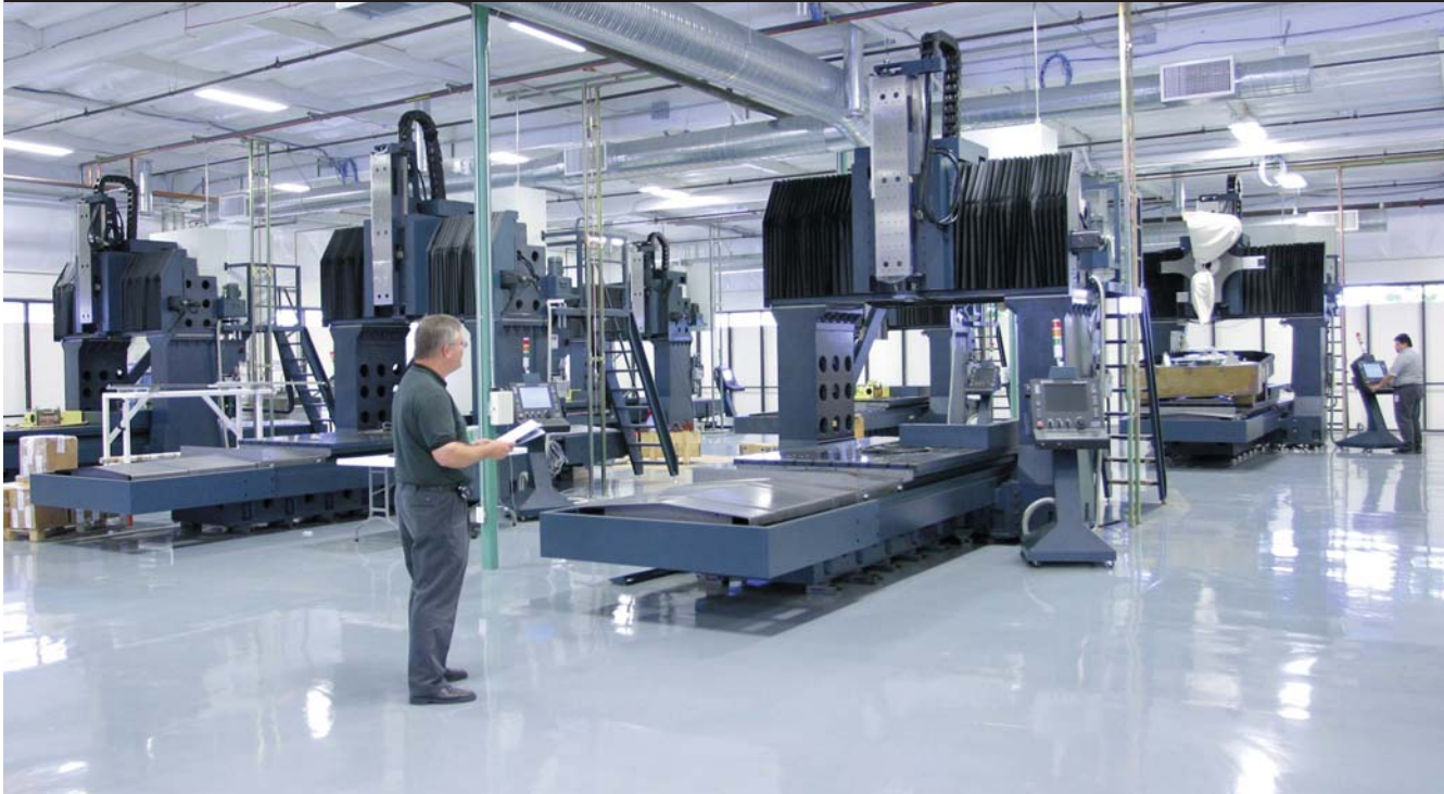
Tracy Peters checks out the installation of 5 of 8 Johnford custom 2600 F machines built to perform slow, super-high precision machining on large, critical lens components for the James Webb space telescope. The 8 machines were redesigned, rebuilt, tested and delivered in a total of 10 months by Taiwanese manufacturer Roundtop Machine Tool. "We considered that a remarkable performance," says Tracy Peters. Tinsley employs 102 people in a 150,000 sq ft facility.
